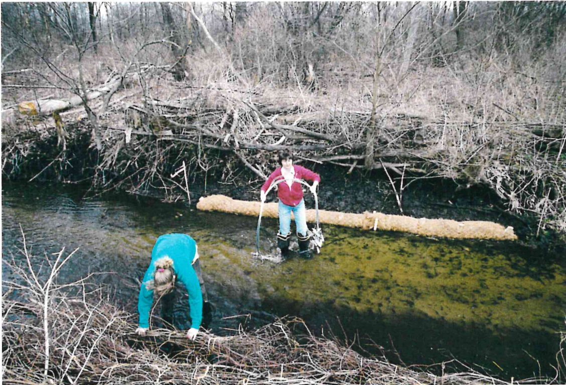
Stacking Fascines for Biolunker
