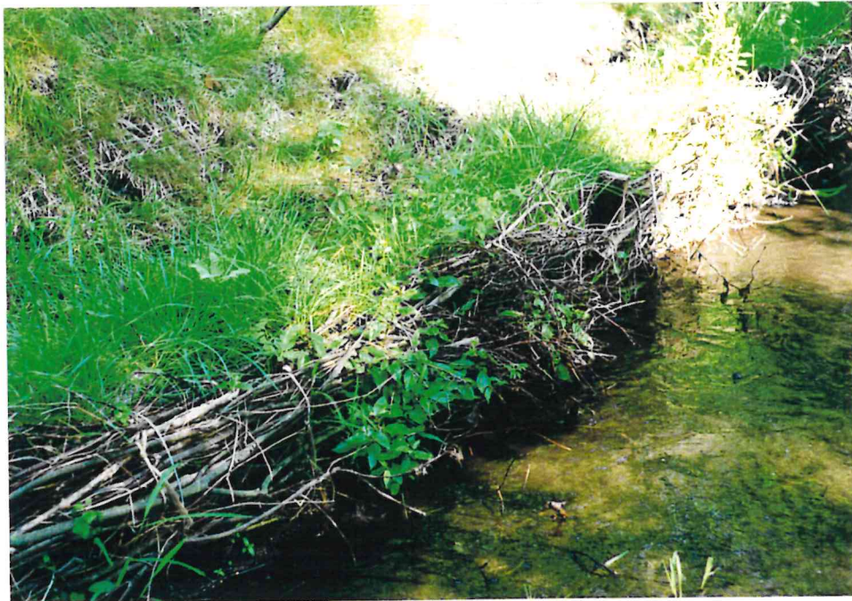
Sprouting Biolunker
