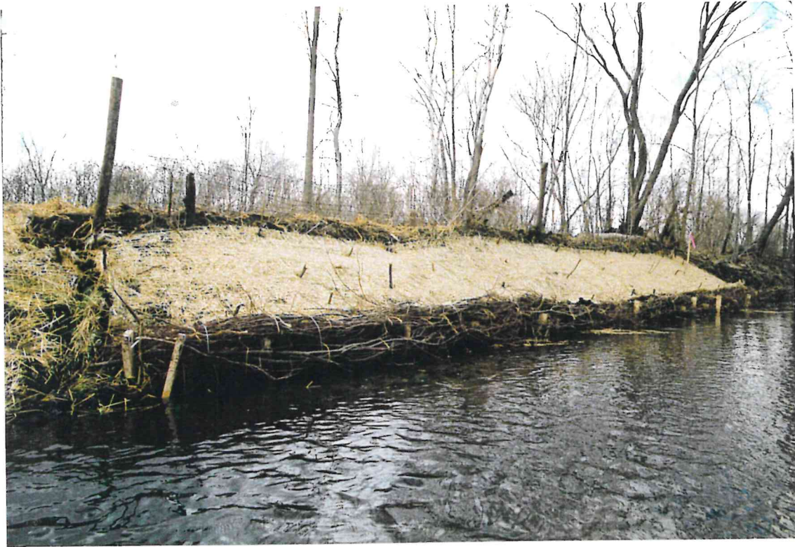
Biolunker After Installation (with seeding above)
