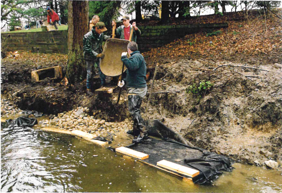
Placing Rock Riprap on Top of Lunkers
