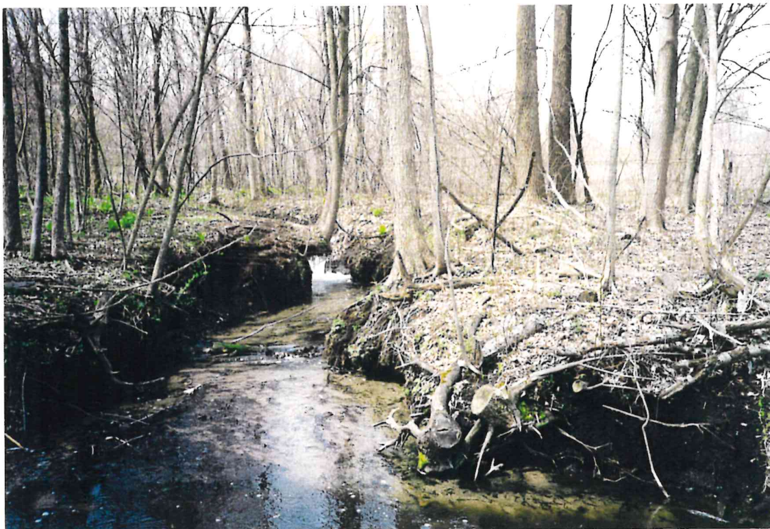
Stream Bank Before Installation of Soil Bioengineering Systems
