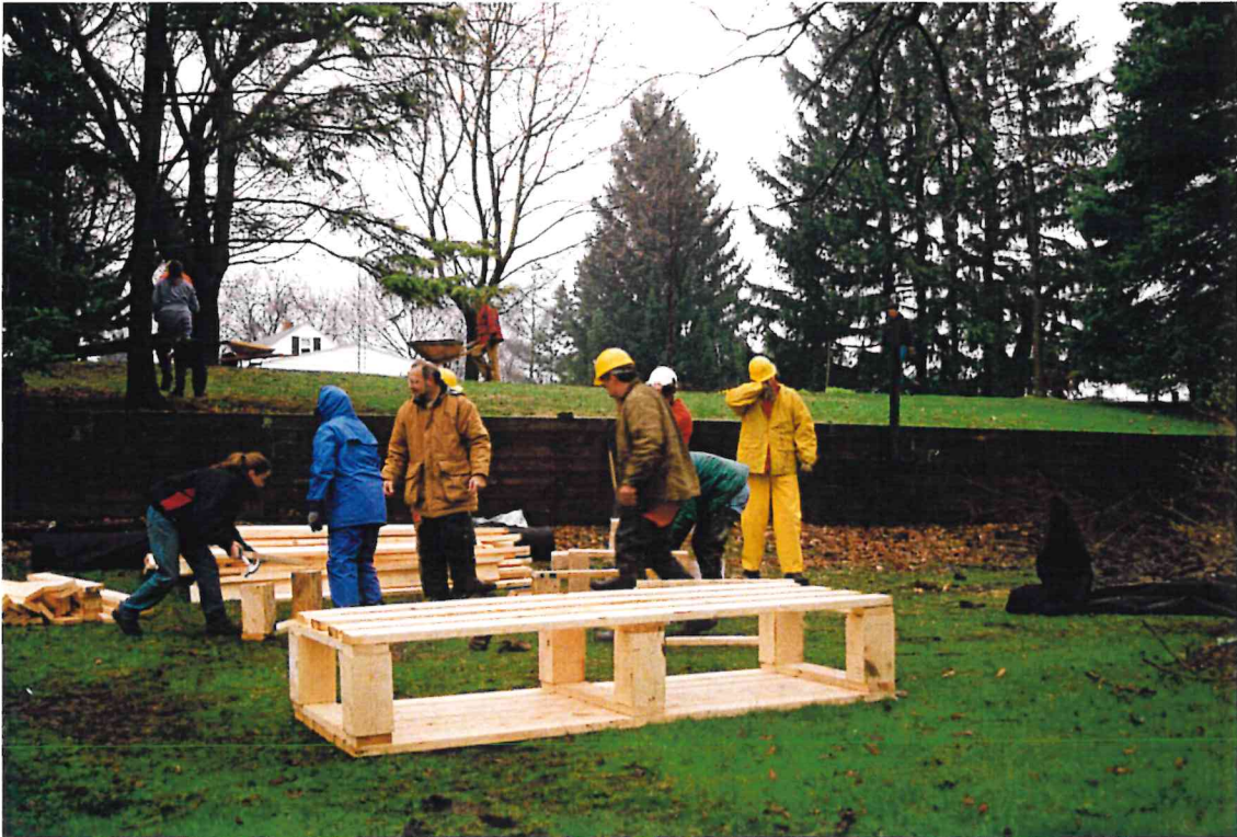
Assembled Lunker Structure
