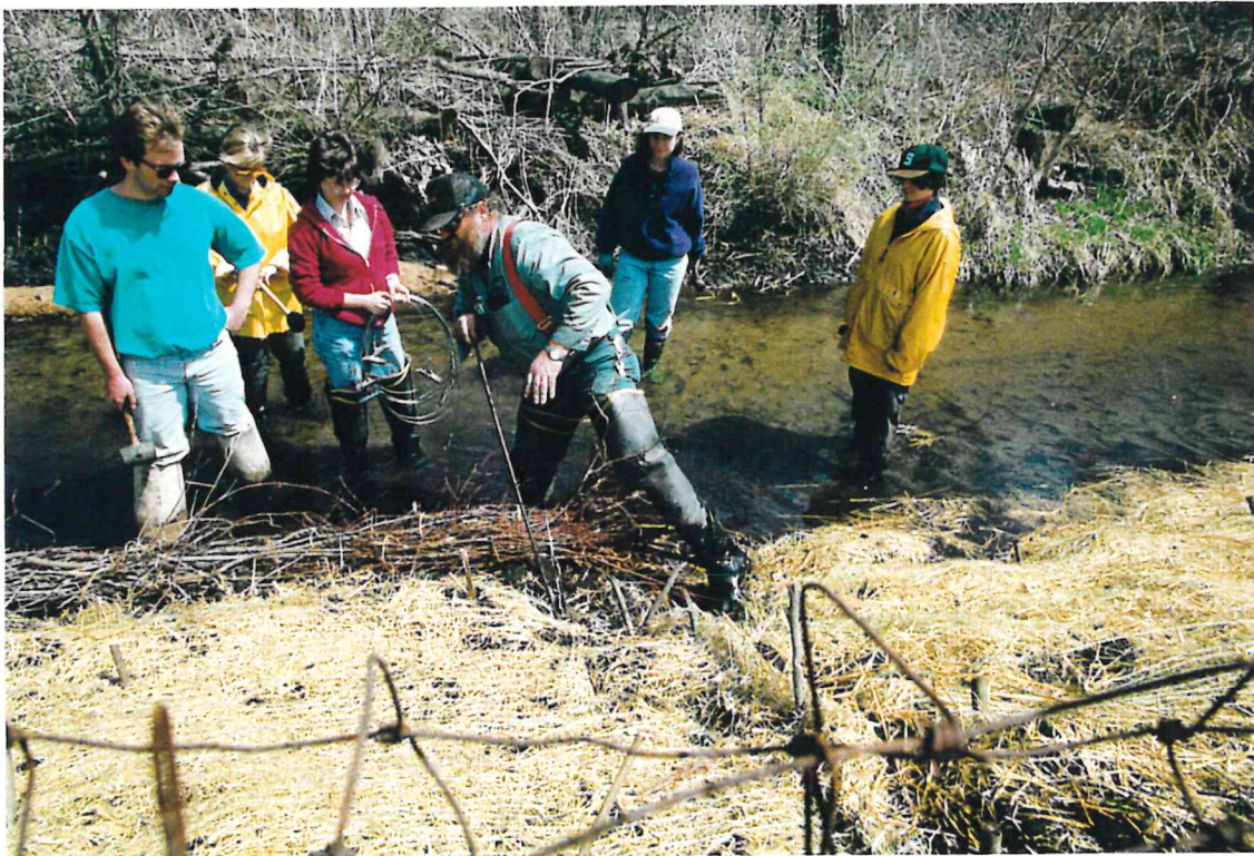
Installation of Duckbill Anchor System for Biolunker
