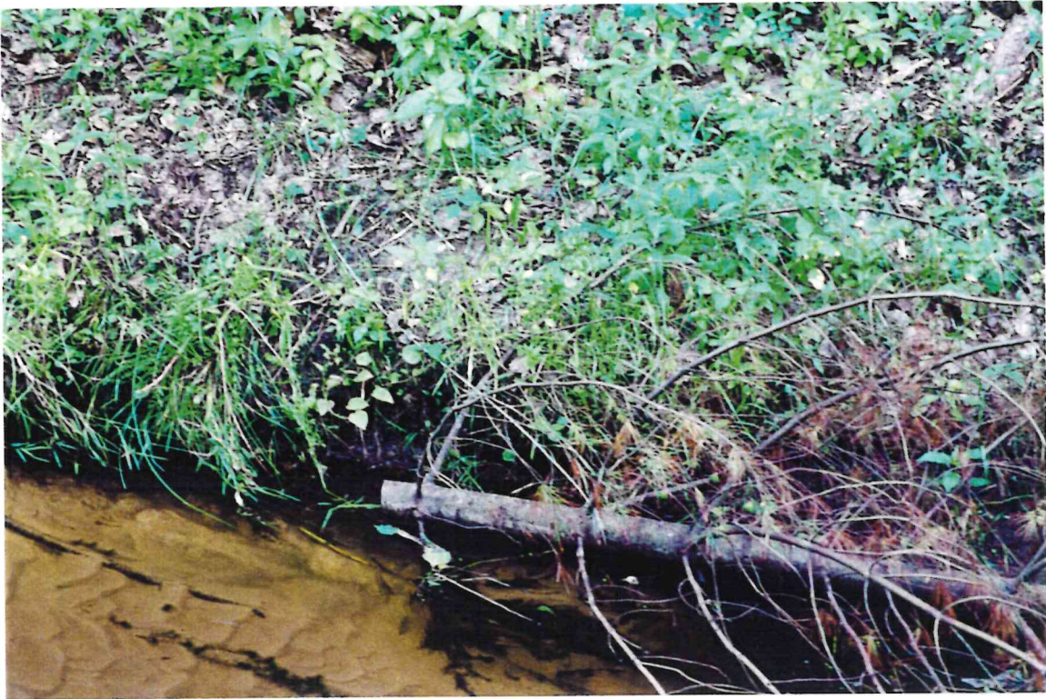
Cable Holding Tree Revetment in Place*
