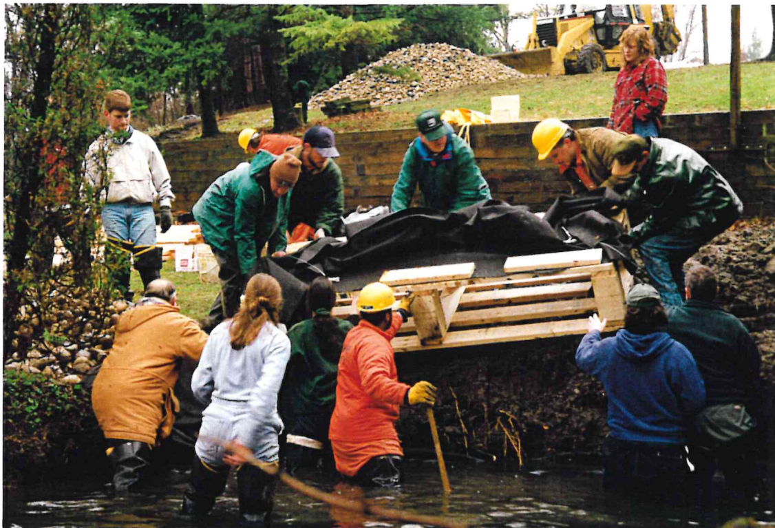
Installation of Lunker Structure
