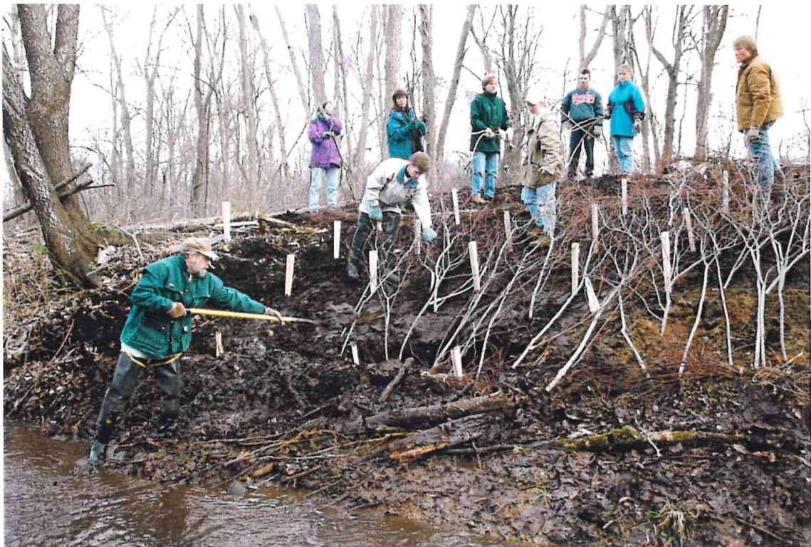
Covering with Dirt
