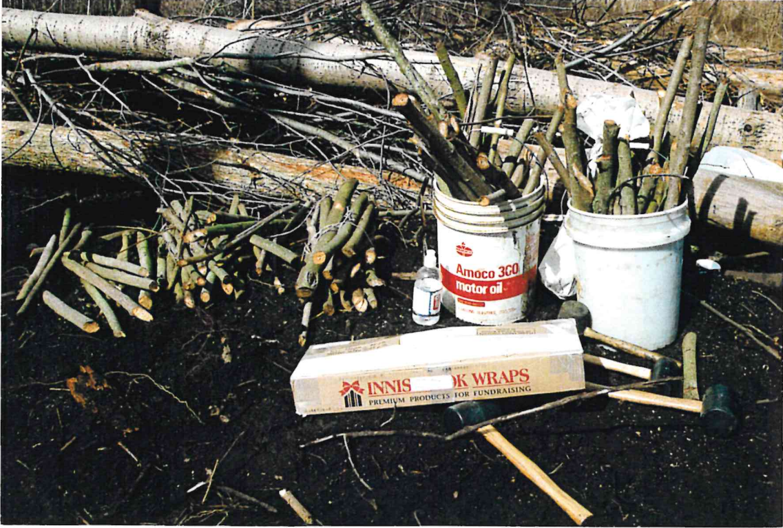
Live Stakes Before Installation
