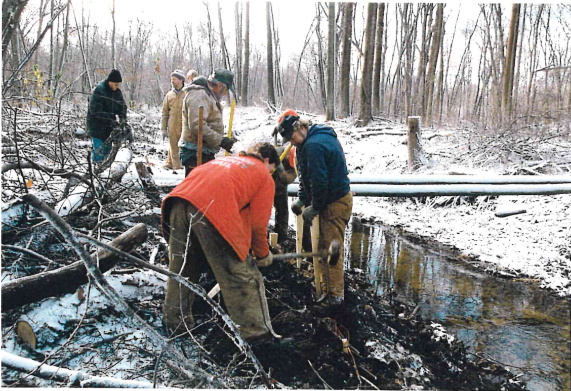
Placing Fascines/Wood Stakes
