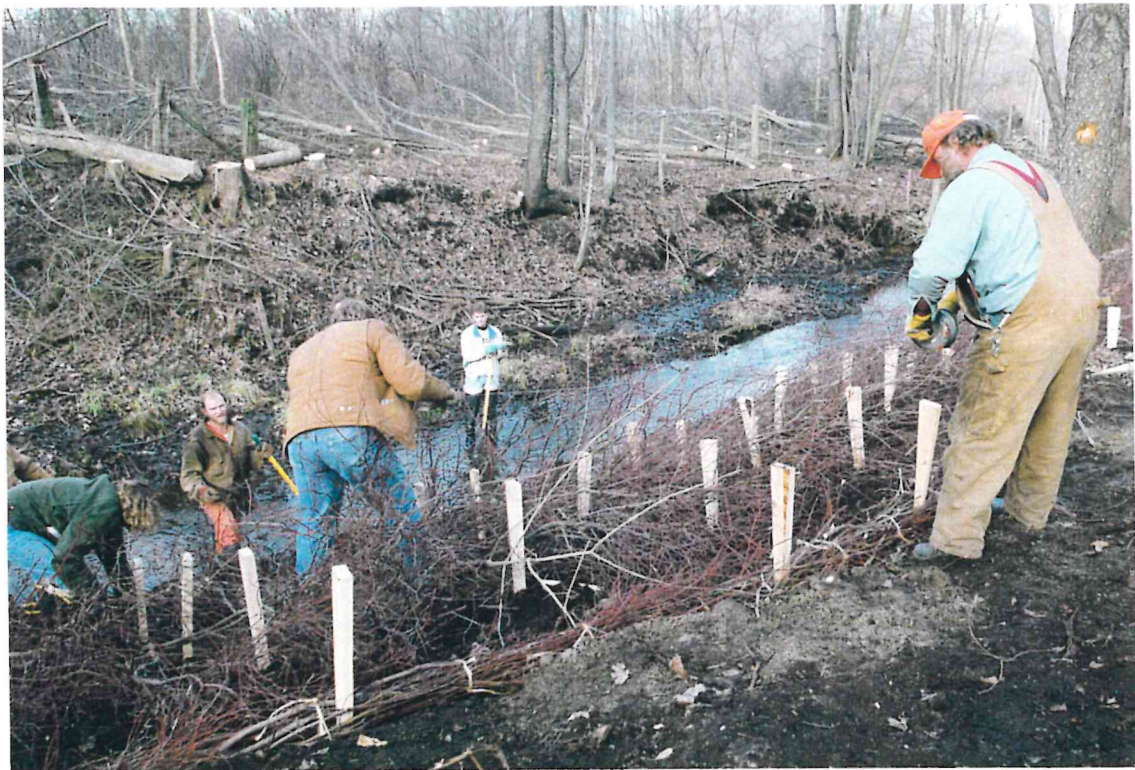
Wiring Brush in Place
