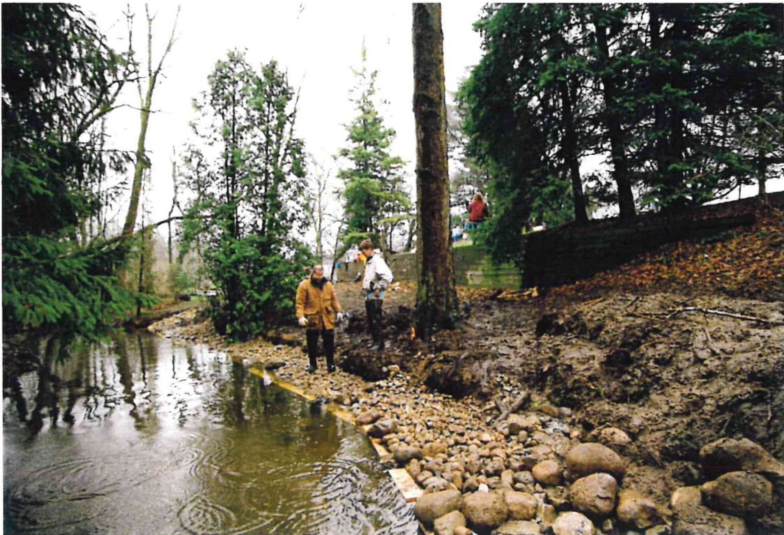
Installed Lunkers
