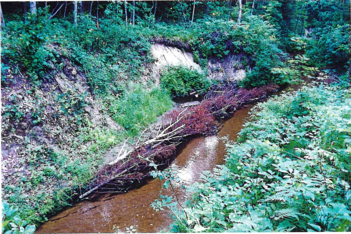
Tree Revetment Installed Along Wheeler Drain*
