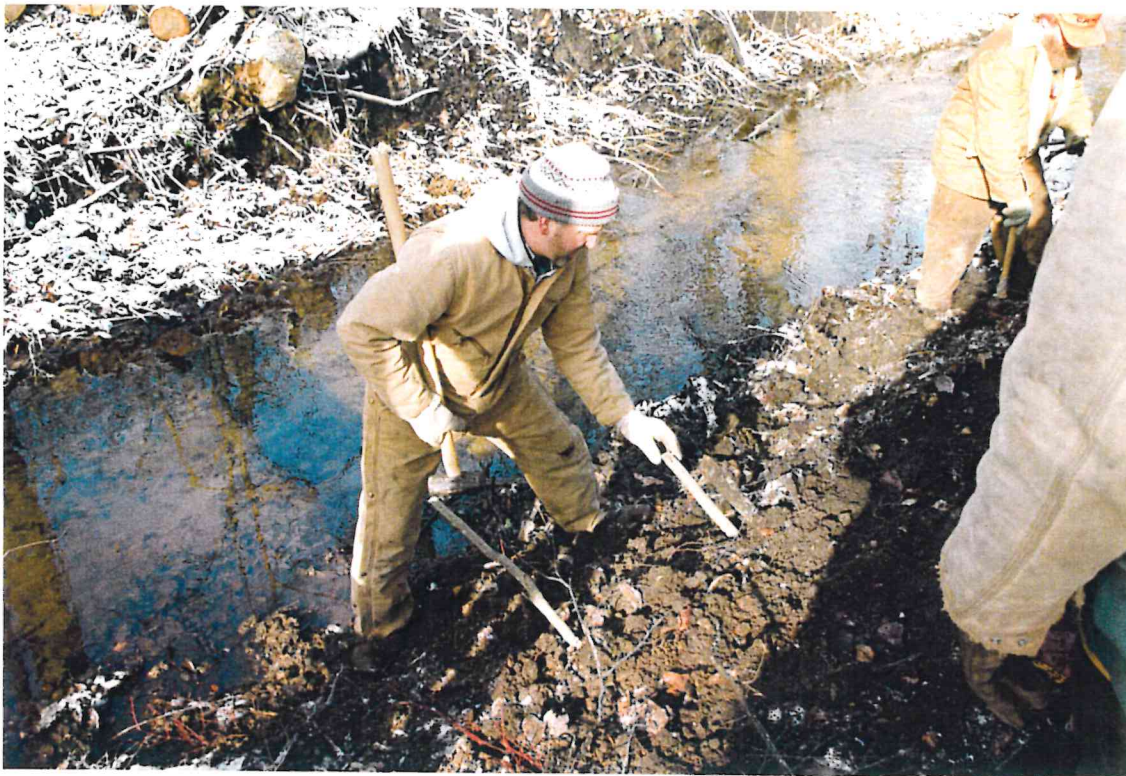
Placing Live Stakes Through Covered Fascine
