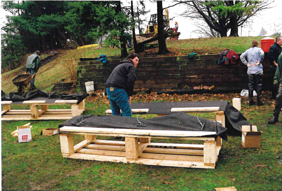
Lunker Structure with Geotextile Fabric and Duckbill Anchors
