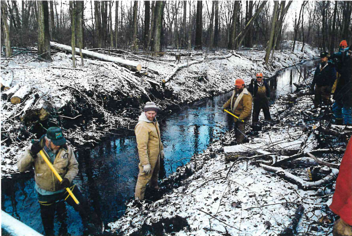
Trench for Fascines
