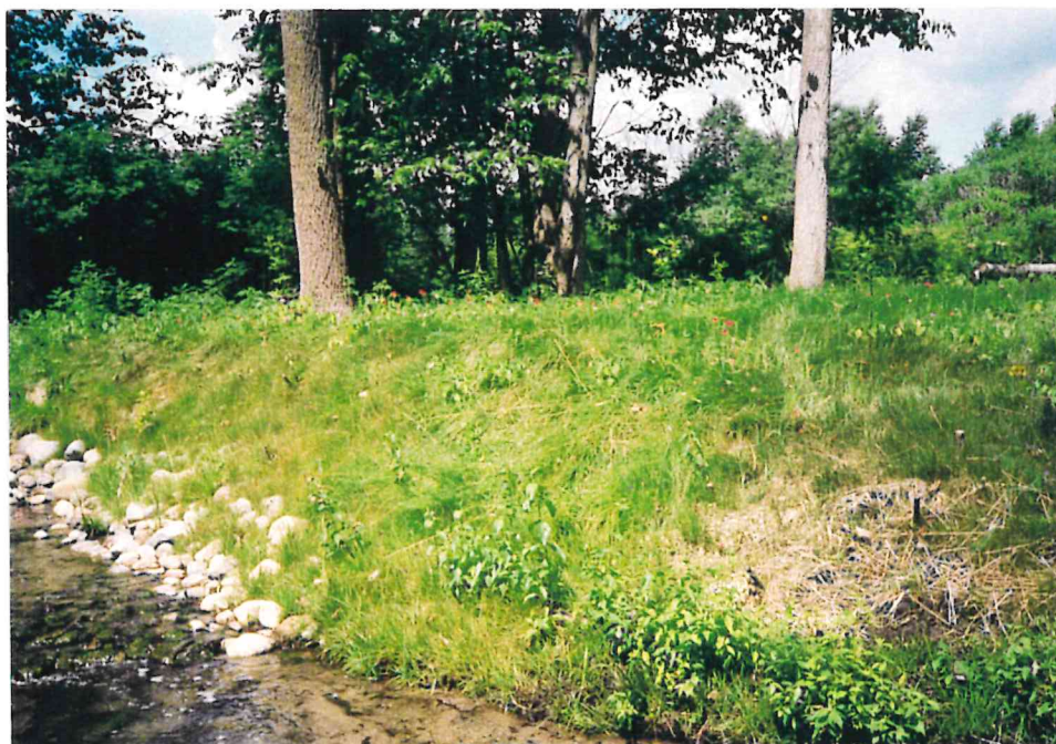
Stream Bank After Installation of Soil Bioengineering Systems
