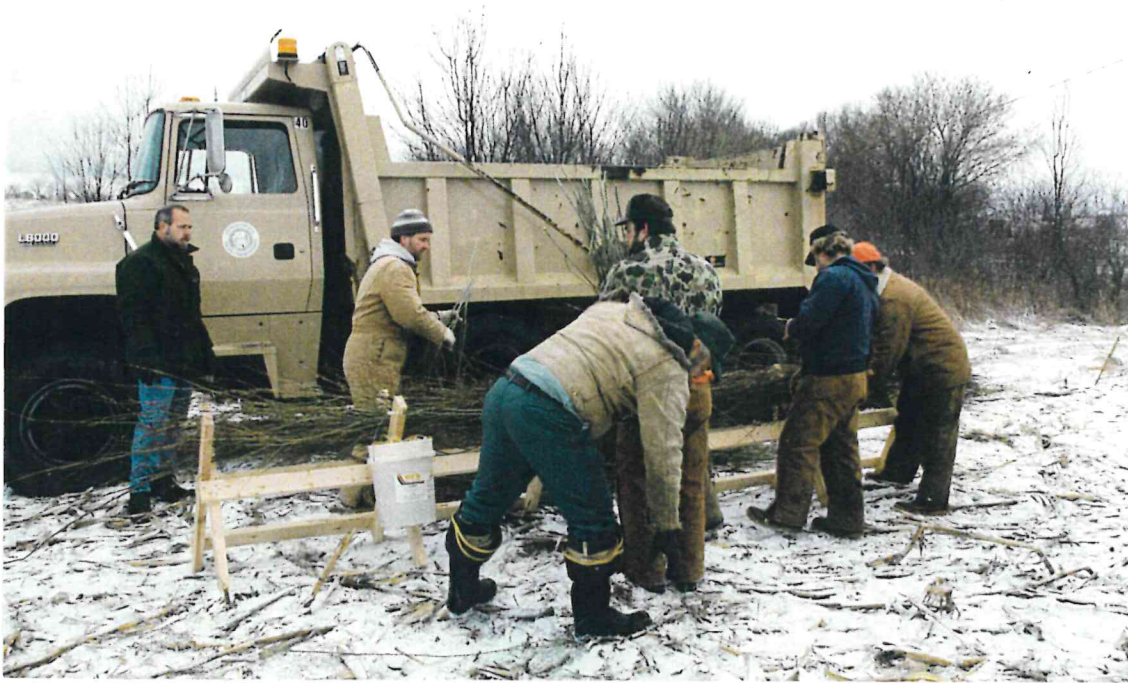
Placing Material in Sawbucks
