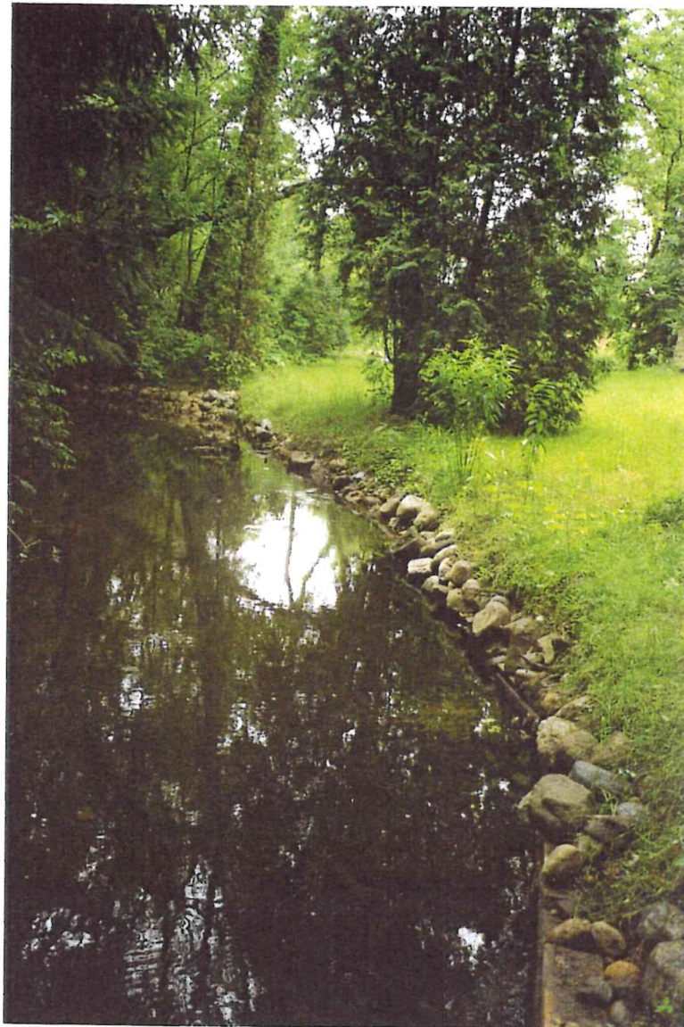
Completed Bank with Grass on Top of Lunkers
