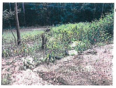
No silt fence installed on the south side of the project site near powerline.
