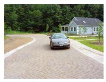
The Pokagonek Edawat Housing Development located in Dowagiac, MI includes the use of 25,000 square feet of interlocking pavers for the primary driving surface.
