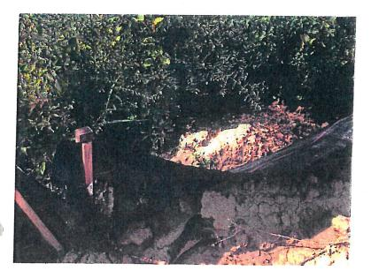
Space in silt fence that needs to be fully closed.
