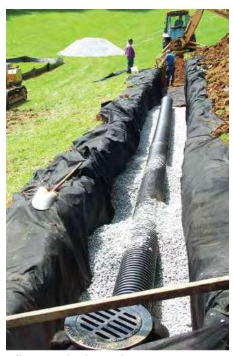
Infiltration trench with geotextile
