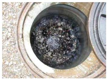
Screening vortex device with floating debris
