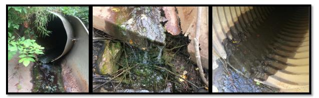
**Figure 9** – Okemos Tile Drain outfall to the Red Cedar River. The photo on the left and center shows algae buildup and corrosion, and was taken during the first round of screening. The photo to the right was taken during follow up screening.
