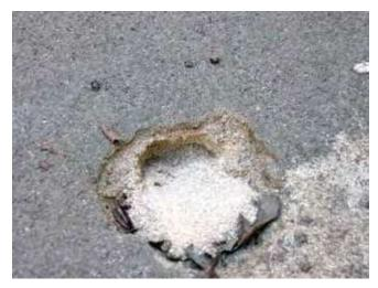
A discolored film on top of a sand filter indicates the need for maintenance
