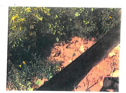
Sediment traveling under silt fence.
