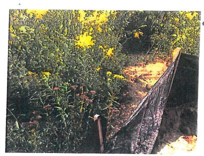
Sediment traveled under silt fence during last rain event. (West side of project site.)
